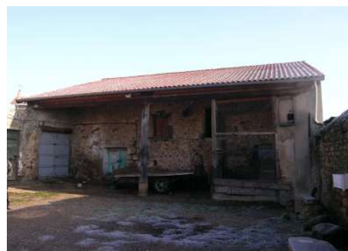
Grange. Route du Large
